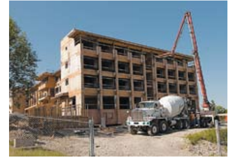
ST. VINCENT'S HEATHER Construction of 68 Assisted Living units is well underway.
